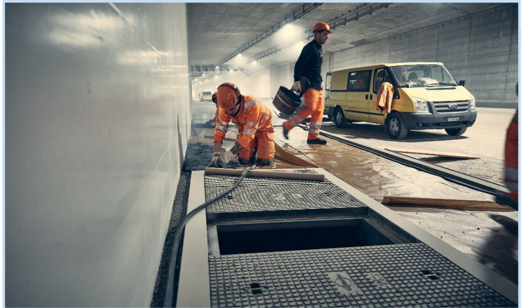
Installation of a cable access shaft with composite material in the Schwamendingen enclosure
