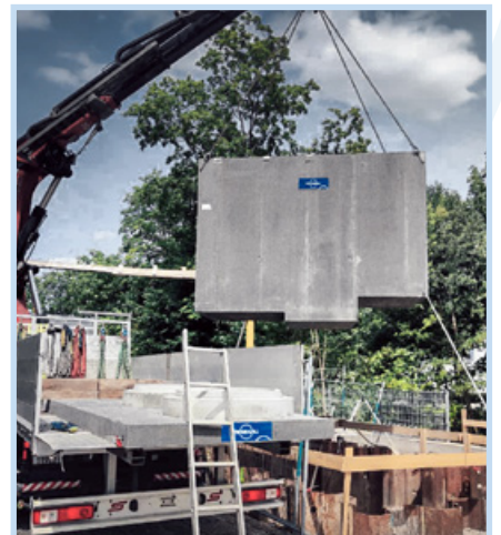
Prefabricated pump shaft, Bottmingen
