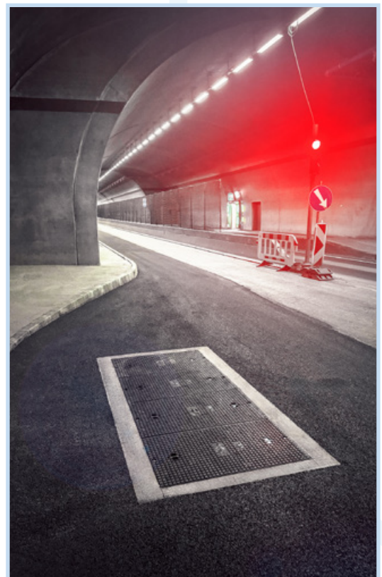
Installation of a cable access shaft with composite material in the Schwamendingen enclosure
